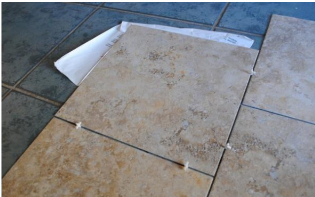
Fig. 1 - Use spacers to maintain the joint width
