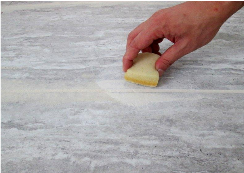
Fig. 3 - Apply light pressure while moving the pad in a circular motion
