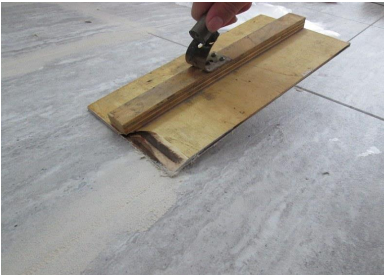
Fig. 2 - Pack the grout into the joints
